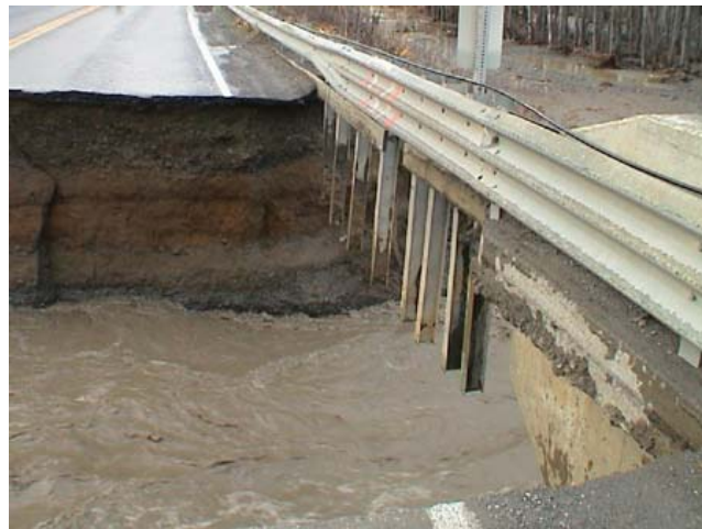
Photo 2: Deep Creek Bridge, Sterling Highway Washout Oct. 2002
