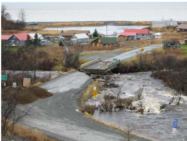
Photo 3: Ninilchik Village Bridge Damage Oct.24-28, 2002
