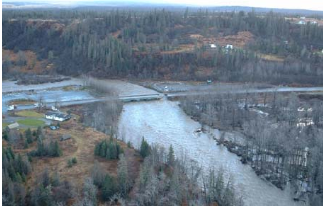
Photo 1: Deep Creek Bridge Washout Oct. 24-28, 2002
